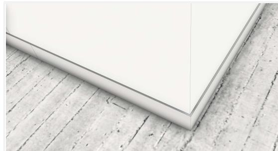
Continue building by connecting each skirting board with the previous one. A new textile tab must be used each time a new set of skirting boards is installed.
