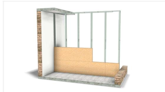
Attach the next panels, using the remainder of the right panel as the start of the first panel. There is no need for the joint to be over a vertical strut.
