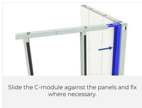
Slide the C-module against the panels and fix where necessary.
