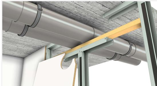
Make a cut-out in the panel. Again, cut a strip off the tongue. Apply it as described above. Finally, slide the panel to the left to lock in place.
