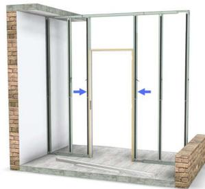
Place the frame between the C-modules and slide the C-modules against the frame.
