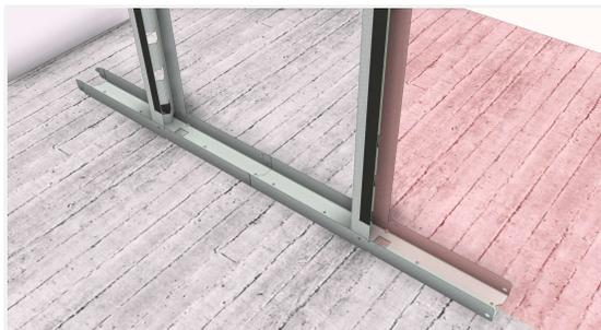
Snap the modules together and centre the end in line with the laser. Fix it.
