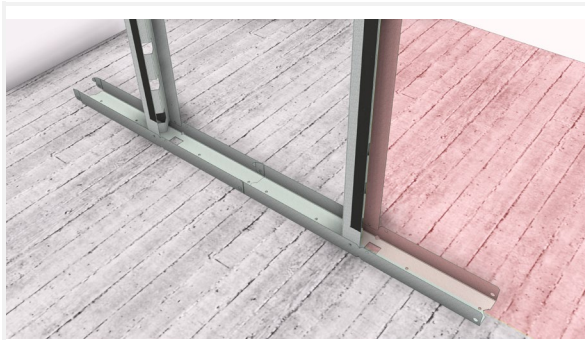
Snap the modules together and centre the end in line with the laser. Fix it.
